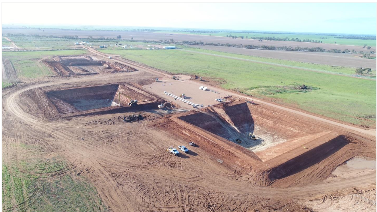
© RayGen Resources Pty Ltd 2021 – Flagship 50 MWh project in construction
