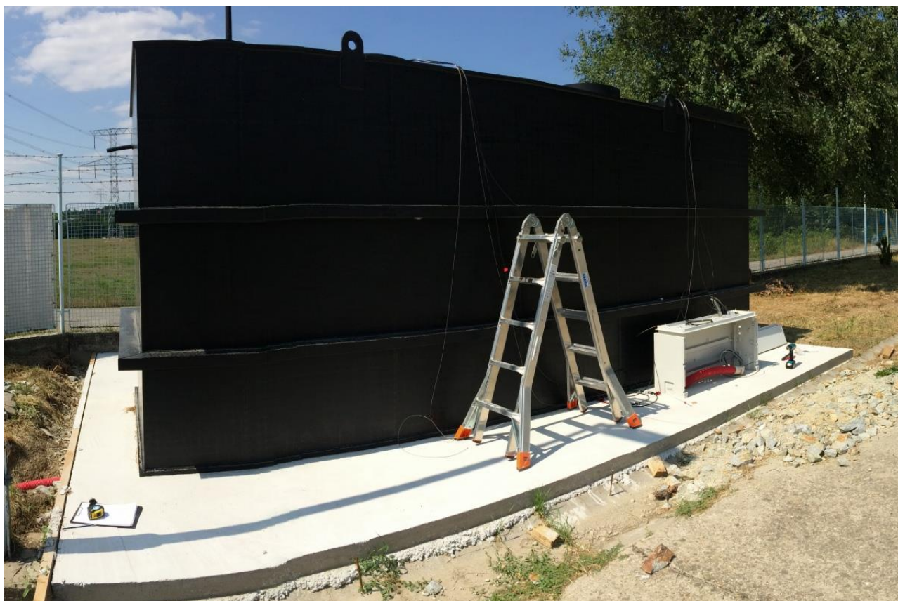
Packaged polypropylene treatment plant for 50–300 equivalent inhabitants (illustrative image, source WYDREX s.r.o.)
